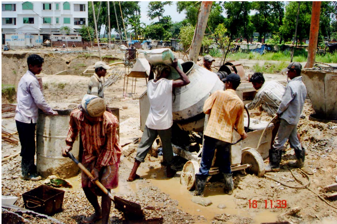
A man engaged in DSE building construction work is pouring brickbats into rolling machine for the final use at DSE building.
