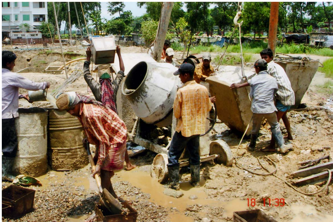
Workers-breaking brickbat, pouring water into drum containing construction materials and carrying materials on the ground of the DSE building (under construction).
