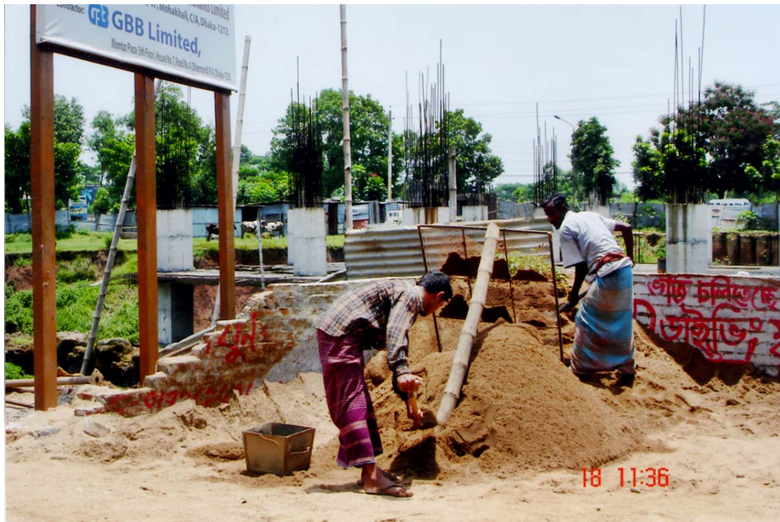
A worker is filtering sand, which will be used for the construction purpose of the 14-storey DSE building.
